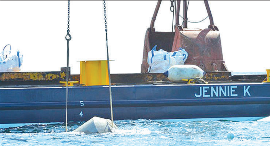
Deploying concrete into the water
